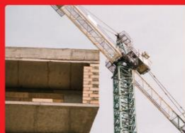
Large tower crane installation
