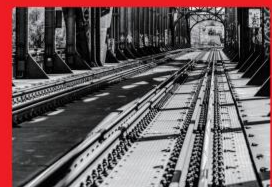
Road and bridge construction
